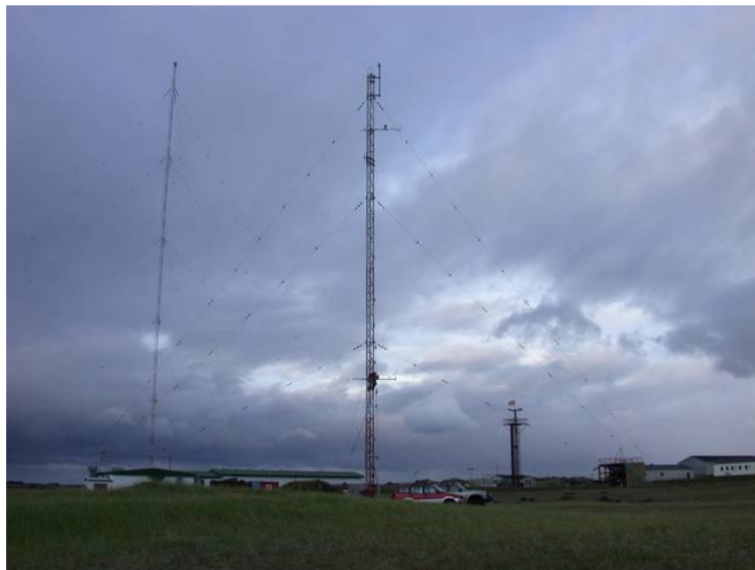
Figure 2. Installation of equipment in one of the two masts at Gufuskálar, W-Iceland in August 2008.
